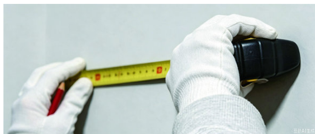
Measure before cutting
