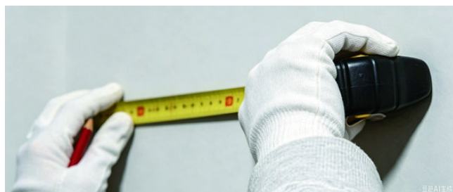
Measure before cutting
